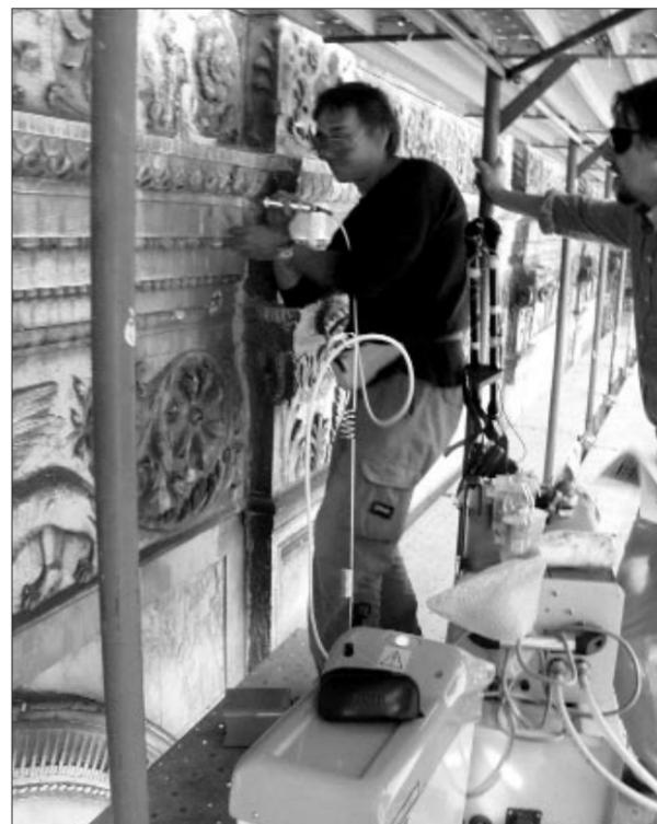
Fig. 6. A modern Laser equipment with optical fibres for the transmission of radiation
