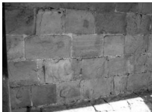
Fig. 4. Natural weathering of water repellent products applied to the Gothic bell tower of the Agrigento Cathedral (Italy). Stone ashblars treated with different products, 5 years after the application. Colour and water absorption by the "contact sponge" method were measured to evaluate the performance and durability of the tested products
