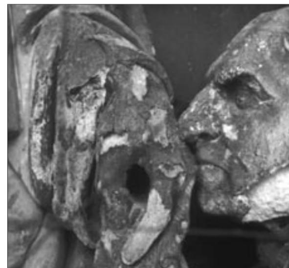
Fig.1 . Venice, Scuola Grande di S. Marco, Lunette by Bartolomeo Bon (16th century): detail of showing the decay of the sculptures, with black crusts and heavy losses of the marble beneath. Photo shot in 1974, before the conservation treatment
